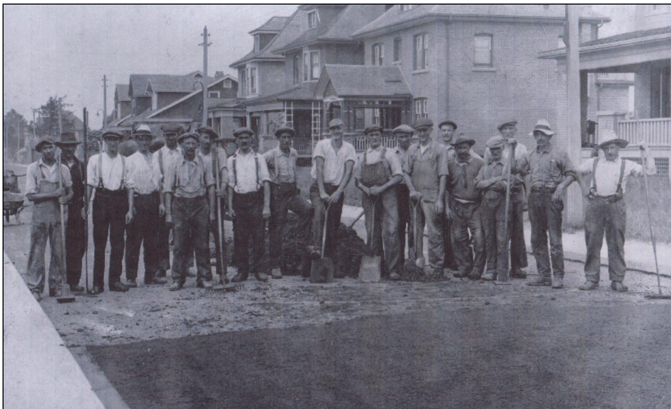
Mark (8 from left) with a work crew paving one of the streets in the 1920s. The men were given jobs by the day because times were tough and there were no jobs to be had.
